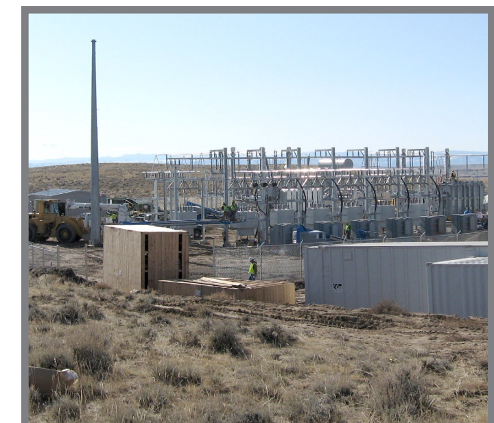
Similar to rural cooperative substations
