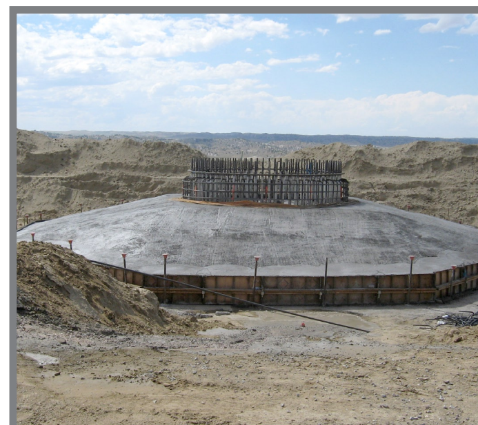
Large mat foundations in shallow excavations
