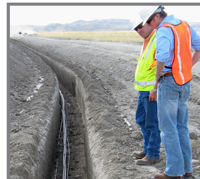
Directly buried in the ground if possible
